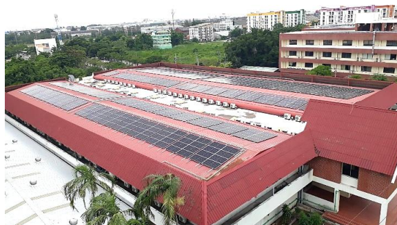
HCU Solar Rooftop Project
