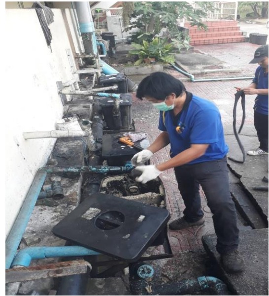
Inspection and cleaning of grease traps
