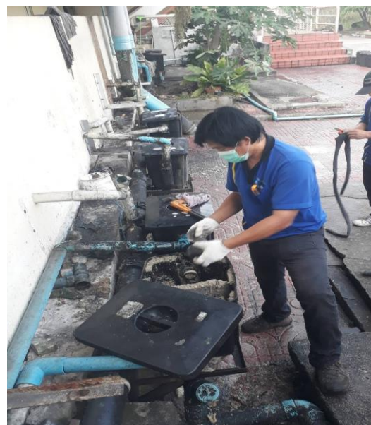
Inspection and cleaning of grease traps
