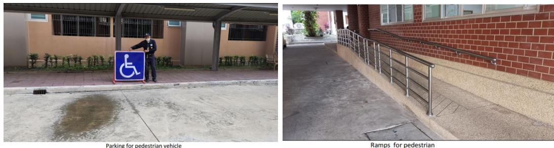
Figure 33 Signage and ramps for the disabled
