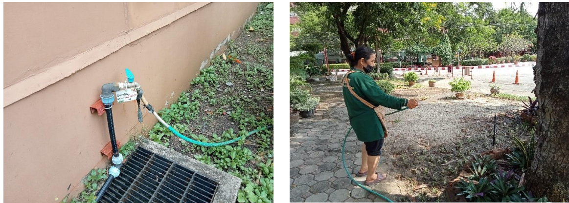
Figure 29 Treated wastewater (effluent) faucet from wastewater treatment system (left) and use of treated recycled water to water plants (right)
