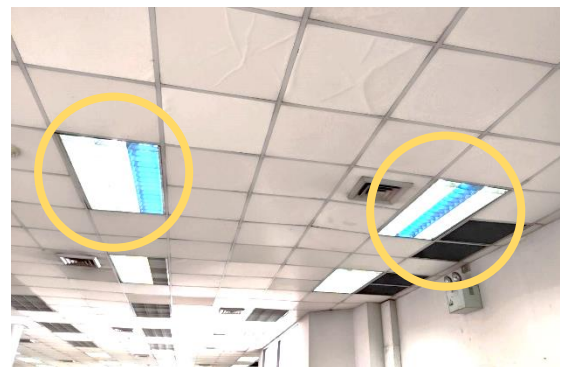
Installation of UV lamps at the waiting area for COVID-19 testing
