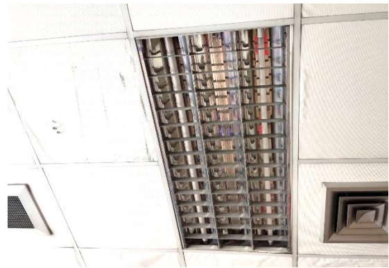
Installation of UV lamps at the COVID-19 testing point
