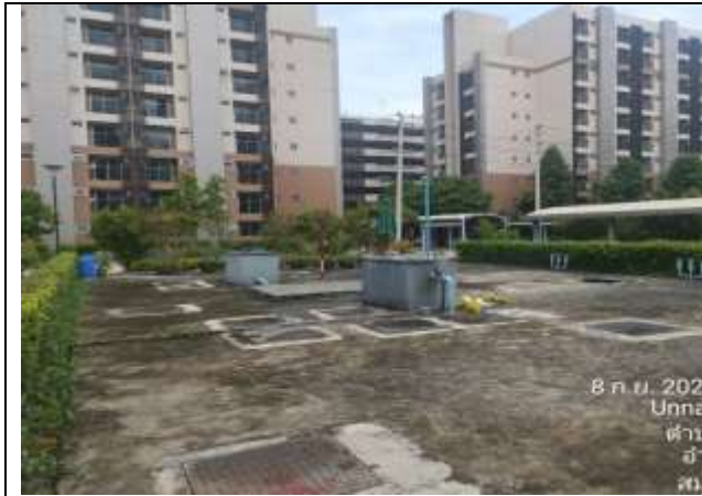
Figure 1. Wastewater Treatment Plants
