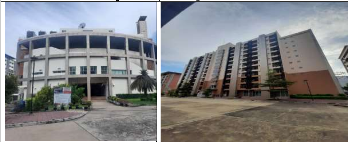
Figure 4. Campus Building Area at HCU2
