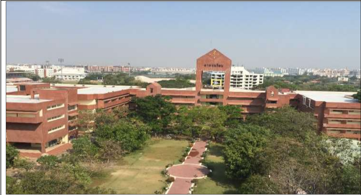
Figure 3. Campus Building Area at HCU1
